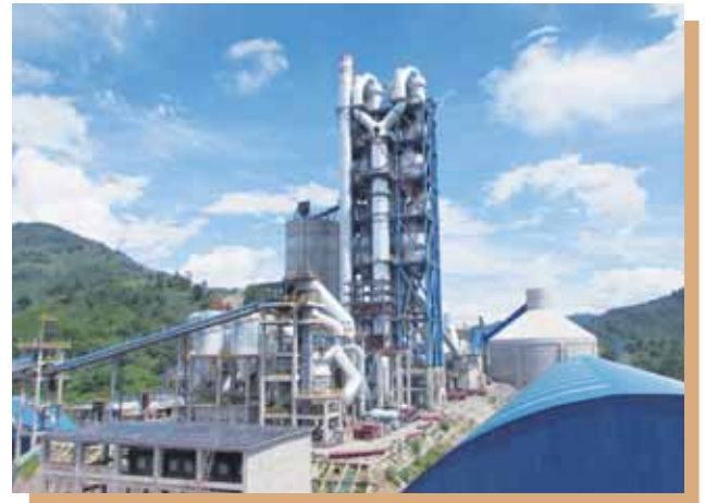
Cement production plant in Puer of Yunnan Province
