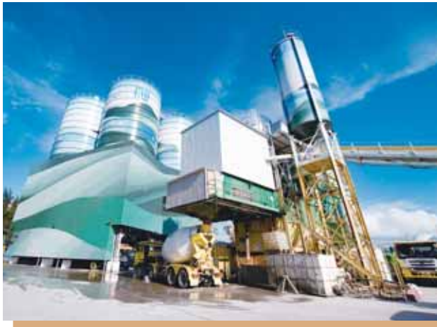
Concrete production plant at Tai Po
